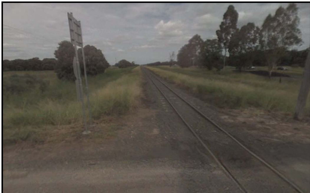
FIGURE 16.4 RAIL LINE NEAR THE STUDY AREA
